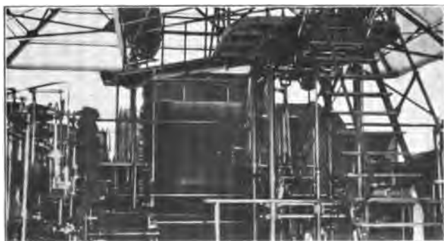
C. NEW HOIST AT FRANKLIN JR. MINE, NO. 1 SHAFT.
